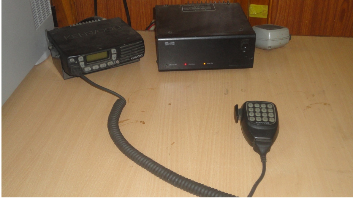
Communication Equipments in DEOC, Viluppuram
