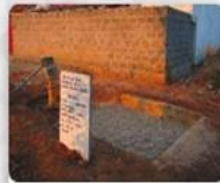
Reuse and recharge structures
