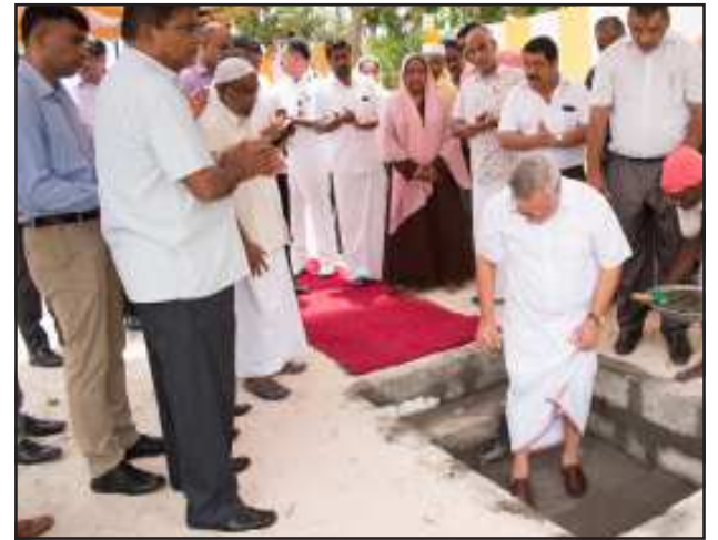
Hon'ble Administrator Shri. Farooq Khan laying foundation stone of Raj Niwas Lakshadweep.
